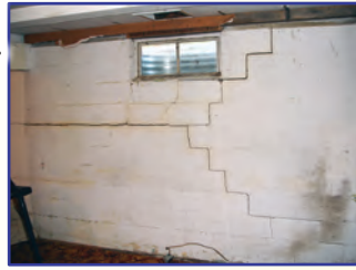
Basement Structural Repairs
